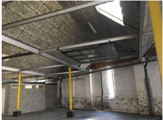
Building and fixing of the grid in the exhibition place (3m x 3m, October 2021)
