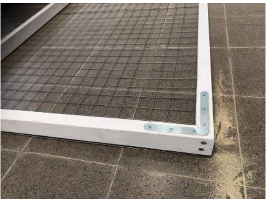
Detail of the flat corner brace at the frame corner. Building of the grid (3m x 3m, March 2023)
